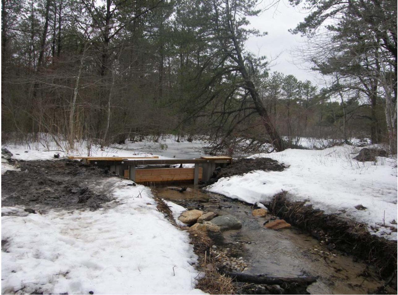
Staundinger's Pond Weir, East Hampton, NY. Installed 2011.
