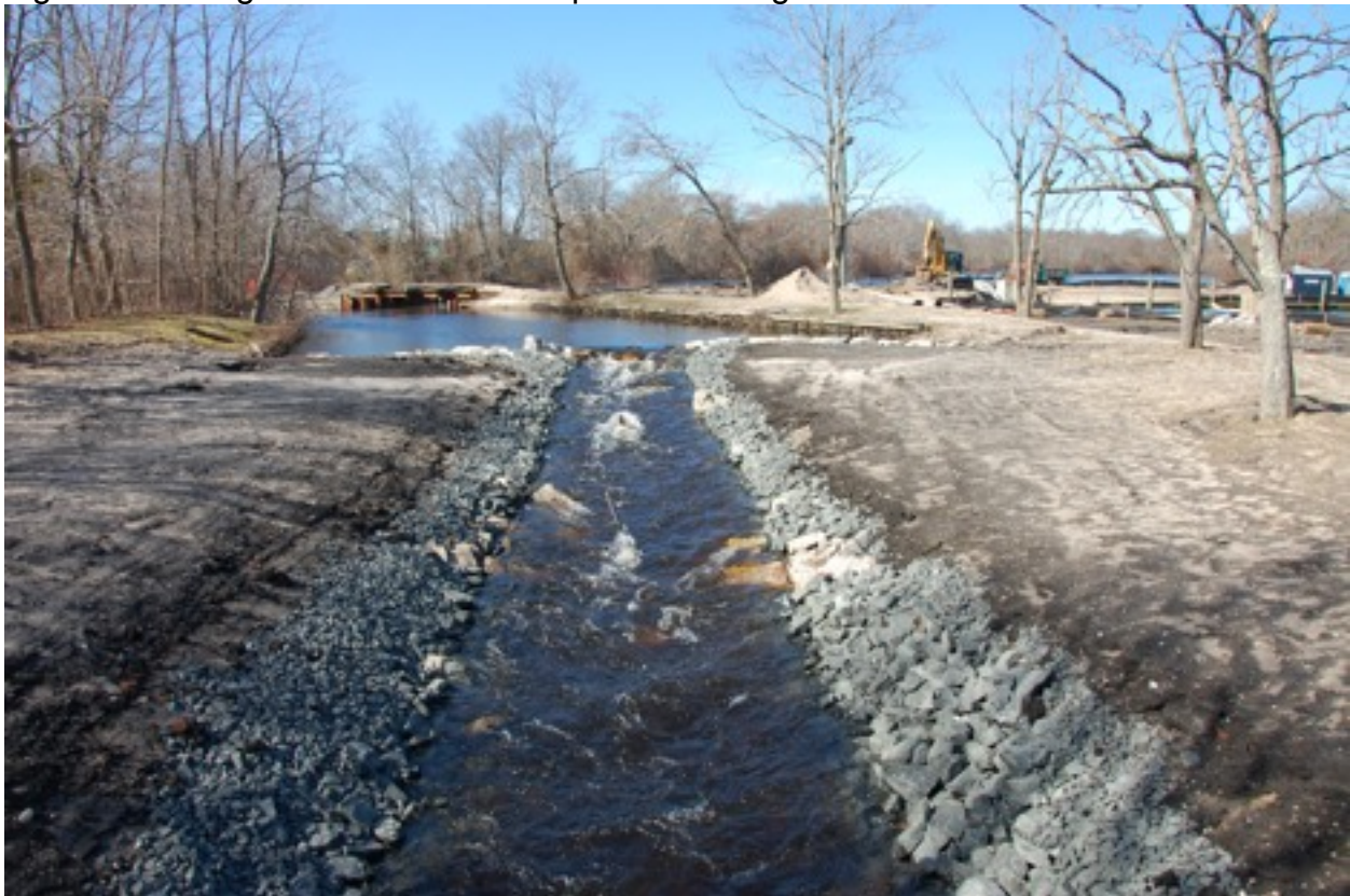
Figure 1. Grangebel Park Rock Ramp Fish Passage.
