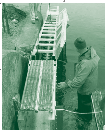
Grangebel Fishway. Photo by Miller Environmental
